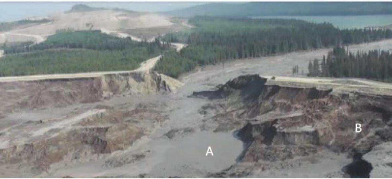
Mount Polley Mine, Likely, BC: spilled 4,500,000 m<sup>3</sup> of tailings<sup>4</sup> with clean up costs of \$200–500 mil.<sup>5</sup> (2014)
